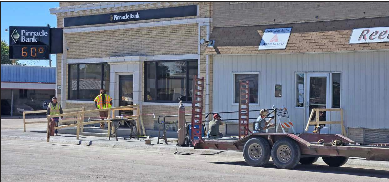
Access to both Pinnacle Bank and Reed’s Food Center has been improved as part of the downtown sidewalk project. To ensure safety, Paulsen, Inc. initially put up temporary handrails. Early this week, a crew of two welders arrived to install the permanent railings. Meanwhile, the main sidewalk crew wrapped up about four and a half weeks of work and left town late last week after completing the vast majority of the project. - Debbie Connelly photo
