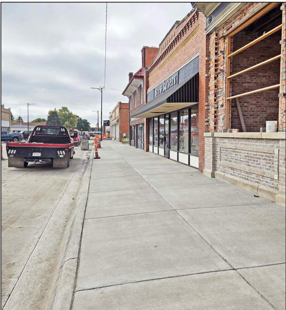
Looking south on the west side of Walnut Street, the downtown sidewalk renovation project was nearing completion as of Monday, with more work to be done at Reed’s Food Center and the bank. With almost total access to the new sidewalks, AEDC Director Cheryl Carson said she has been receiving good feedback from residents, who are enjoying the safer walkway. - Debbie Connelly photo
