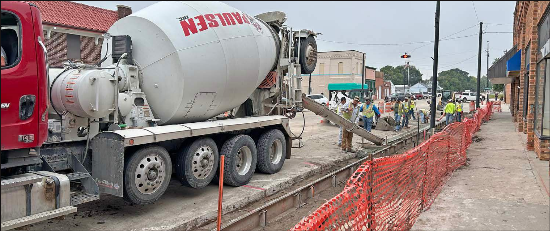
It was noisy and busy on the east side of Arnold's main street last week, as contractor Paulsen, Inc. began the much anticipated downtown sidewalk renovation project. Starting on Tuesday, the large crew was making pretty quick work out of tearing out a full-length section of old curb and a portion of the sidewalk and setting forms. By Thursday morning, the workers were pouring and screeding the curb down the block. The Sentinel will continue keeping our readers up to date with photos as more progress is made.
