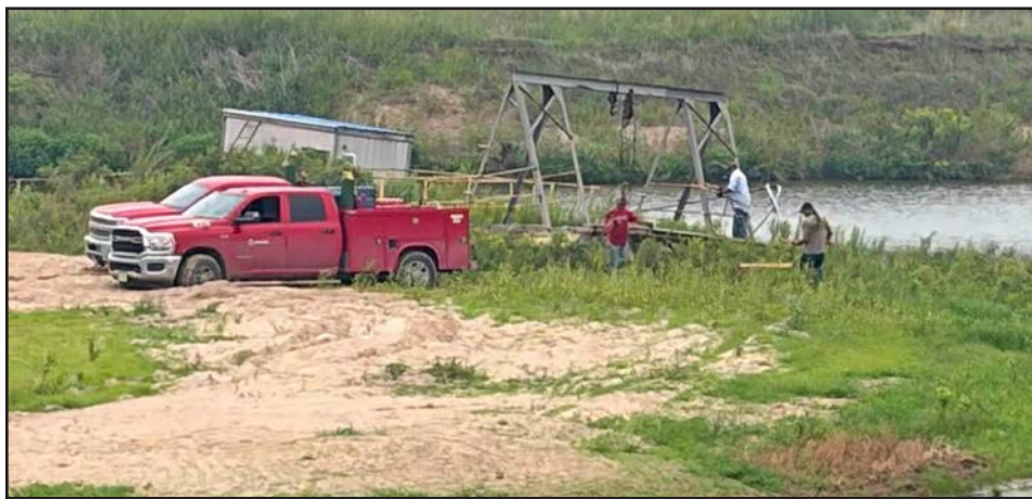
Crews get ready to remove the A-frame from the Beshaler Gravel pit site.
