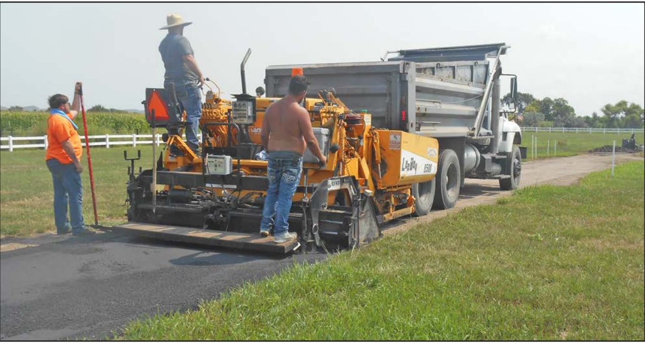
Crews were resurfacing the old roads at the Arnold cemetery on August 7.
