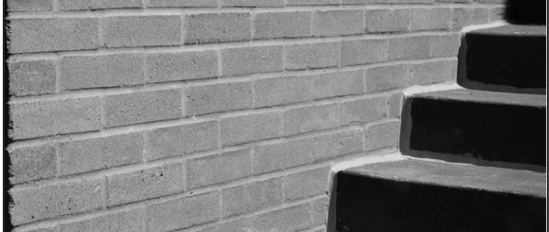
A skilled worker fills cracks with mortar on the library's exterior during the tuckpointing process. Below shows the finished product and the newly caulked steps. (Jessica Tickle photo)
