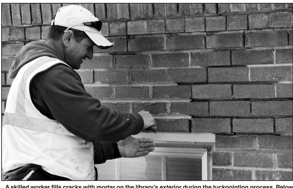
A skilled worker fills cracks with mortar on the library's exterior during the tuckpointing process. Below shows the finished product and the newly caulked steps. (Jessica Tickle photo)
