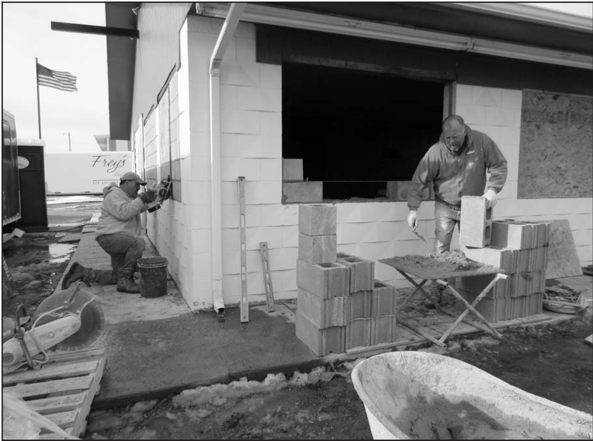
Masons block up existing windows in the former Cardinal Inn, as part of a major remodeling project that started a few weeks ago. The building will be the new home of Arnold Insurance Agency, with completion scheduled in the spring. (Janet Larreau photo)
