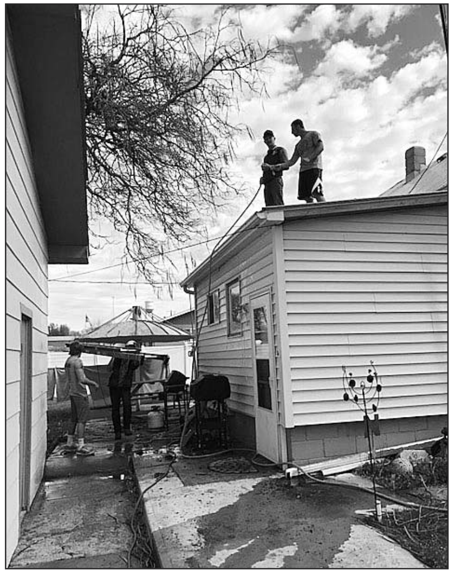
High school students Cade Connell and Blake Schwarz were found on the roof of a residence cleaning out gutters during the community clean-up. Volunteers lent a hand to several residents who needed help with spring cleaning. (Fallon Gibson photos)
