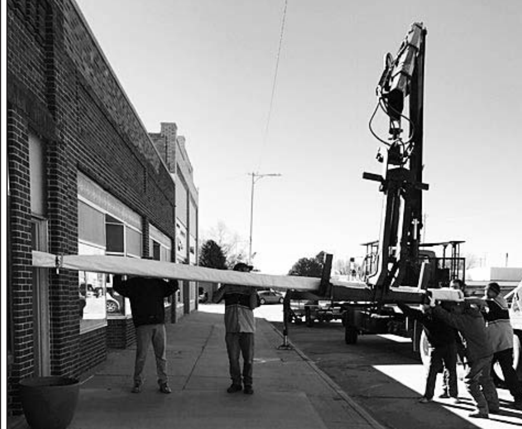
The delivery of a 750 pound beam by Bloedorn Lumber of North Platte to The Sentinel office last week drew a lot of attention on the street and willing volunteers to help guide the beam into the building—including a crew from Forrester's Dodge City that wasted no time in coming to offer help. The beam will be installed to shore the sagging roof up as part of the major renovation process. Meanwhile, The Sentinel office is temporarily located in Hotel Custer. (Fallon Gibson photo)
