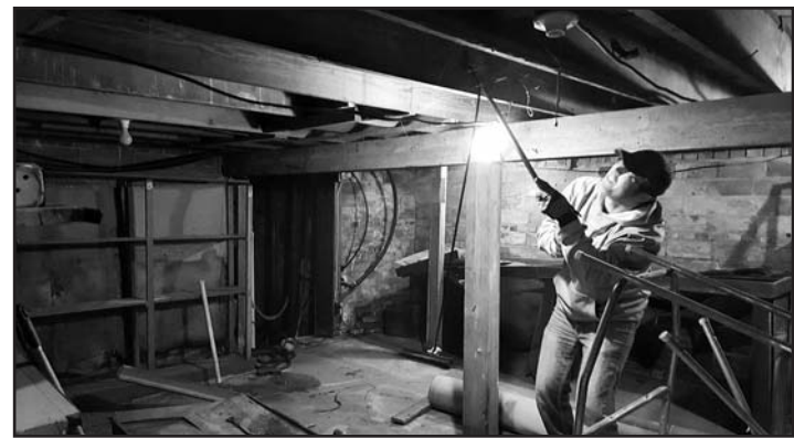
Justin Strasburg works on the second level of the building.
